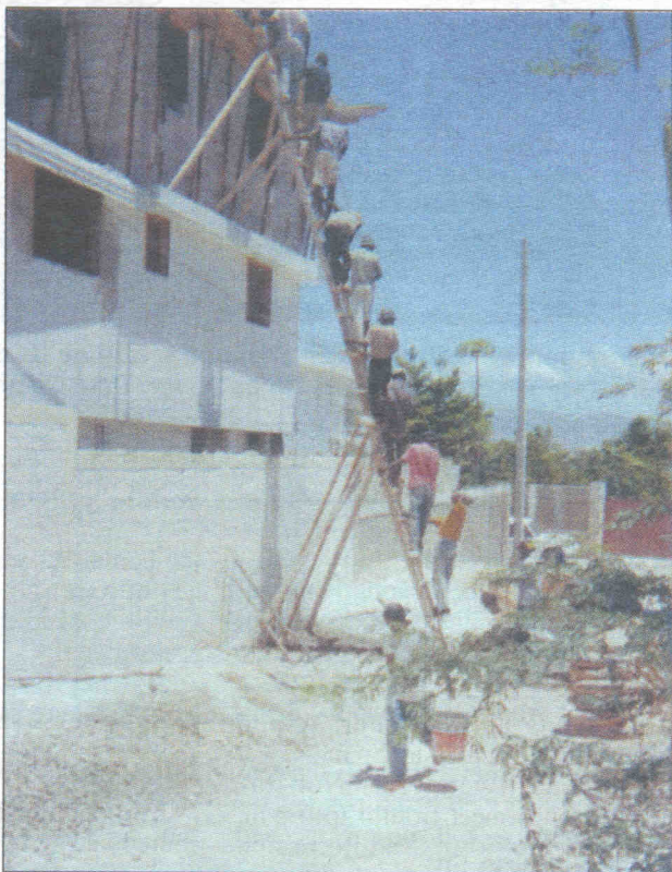
A crew working for the Aspen-based Mercy and Sharing Foundation in Port-au-Prince, Haiti, builds a clinic the old-fashioned way with manpower hauling concrete up a ladder. Photo courtesy Susie Krabacher.
